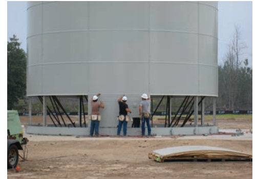
Standpipe - jacked from grade level
