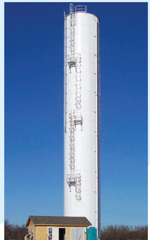
Bolted RTP Standpipe
