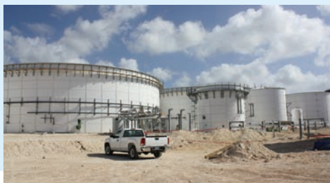
Water & Wastewater Facility
