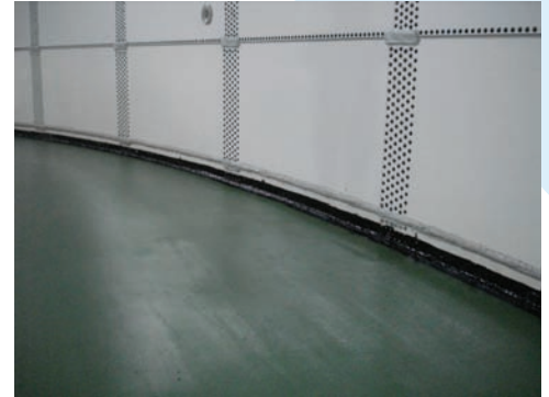
XL Municipal Water Storage Interior Base Setting Ring with Concrete Bottom
