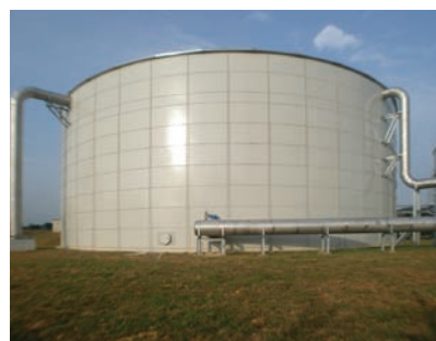
Potable Water Storage
