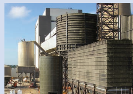
Bolted RTP, Field-weld & Hybrid Tank Construction
